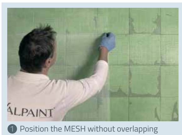
A 74K PV 127 FIBRE-GLASS MESH
