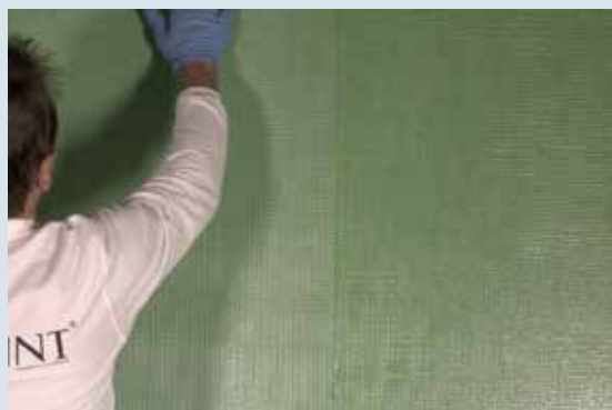
③ Position the MESH without overlapping
