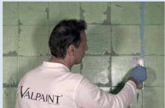
10 Fill the grout lines and any holes in the surface
