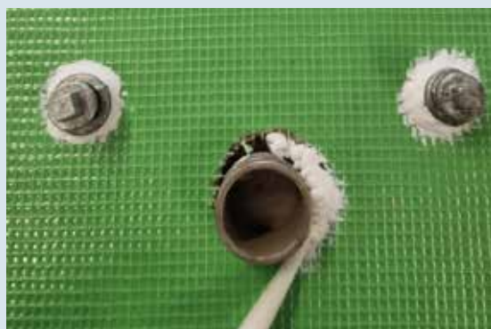
① Applying SIGILLANTE SG15
