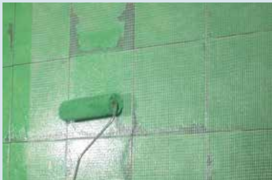
9 With roller pass it over the mesh to make it adhere
