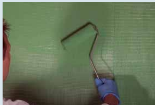
④ With roller pass it over the mesh to make it adhere
