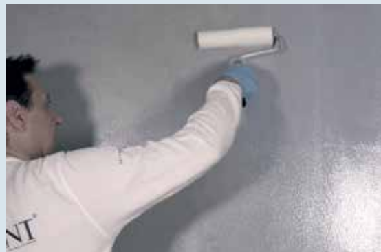
④ To apply 1° coat of TOP COAT LUCIDO o OPACO
