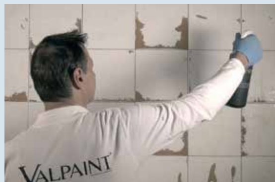
4 Spraying it all over the surface the PROMOTORE
