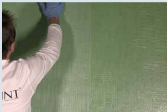
3 Position the MESH without overlapping
