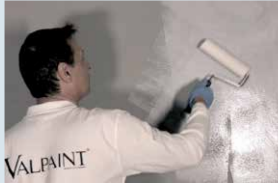
② To apply a thin layer of OTTURAPORI OTB + CT45
