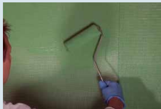
4 Whit roller pass it over the mesh to make it adhere
