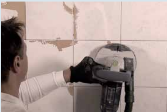
1 Grind and level uneven ceramic
