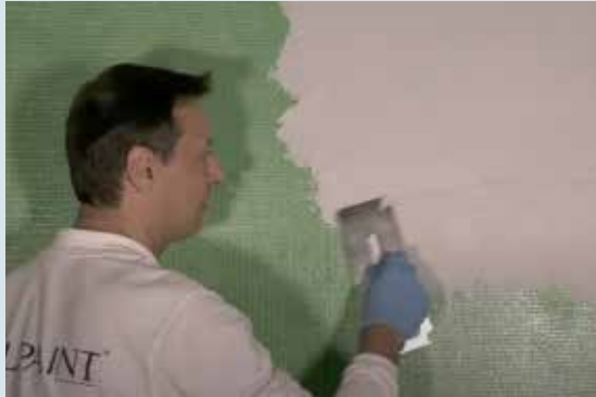
1 Apply a skim coat of METEORE 14 MEDIO
