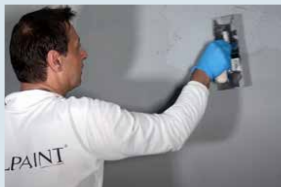
④ Applying a second coat of METEORE 14
