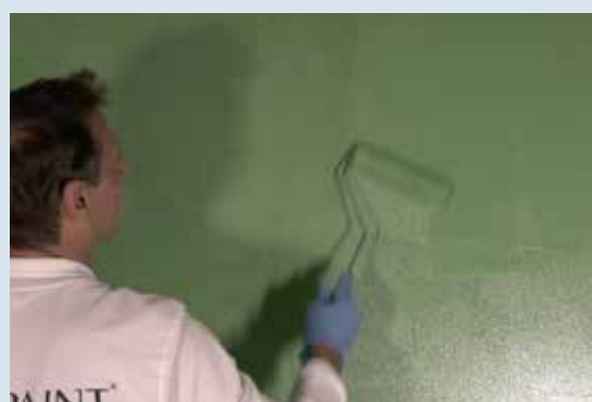
2 2° coat of PRIMER AZ+CT10 not diluted with PROMOTORE
