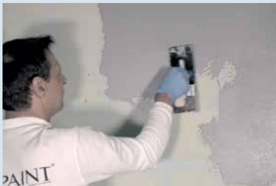
① Apply a first coat of METEORE 14 MEDIO
