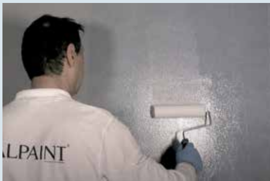
● apply 2° coat of TOP COAT LUCIDO o OPACO
