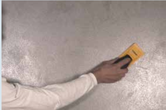
① Clean the surface of any lumps and dust
