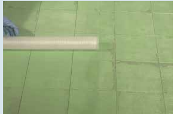
8 Position the MESH without overlapping
